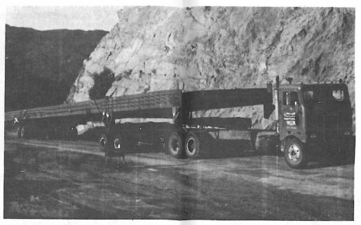
Here is one of those huge steel girders rounding Deadman's Curve at 8 a.m. Tuesday, holding up traffic for only about 10 minutes. They are being placed on supports at the Sweetwater bridge. They are 10 to 13 feet wide, up to 125' long, weigh many tons. See photos Aug. 22 & Sept. 12.
